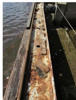
We performed an evaluation of the existing steel coating systems and conducted nondestructive thickness measurements of steel components to identify the severity of corrosion. Drilled core samples and steel coupon samples were obtained for laboratory testing.
