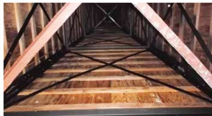
Interior view of spire sheathing construction around the braced steel framing.
