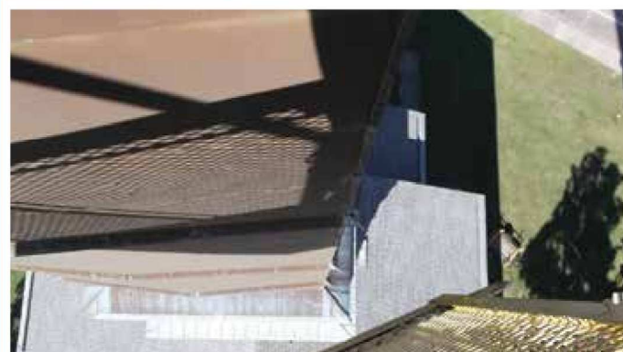
View looking down deformed spire cladding from crane basket.
