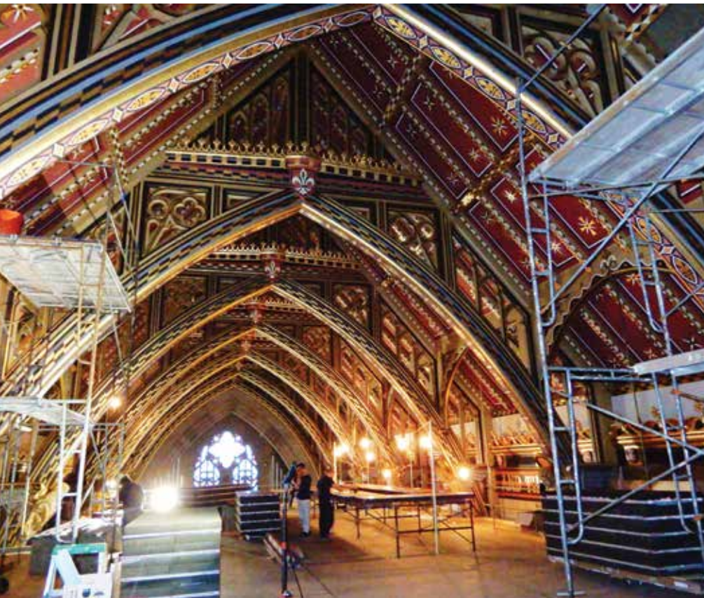
Painting of prefabricated panels on the scaffold near the ceiling.
