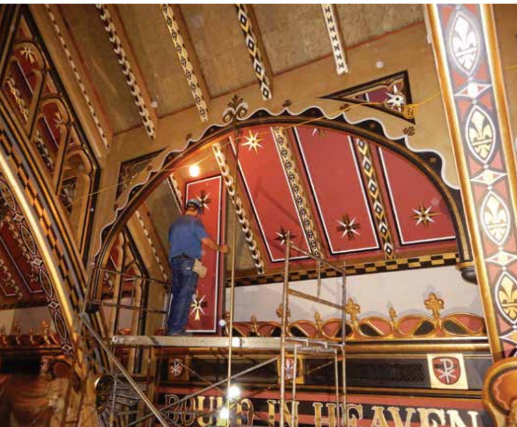
Panel installation in progress.
