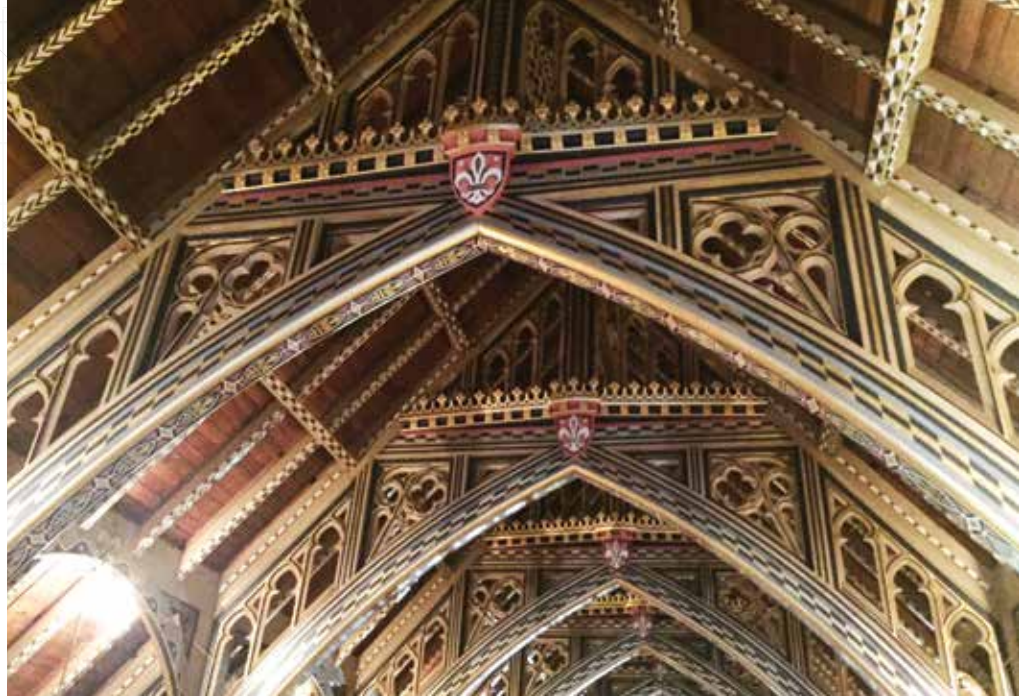
Exposed wood decking and decoratively painted wood framing.
