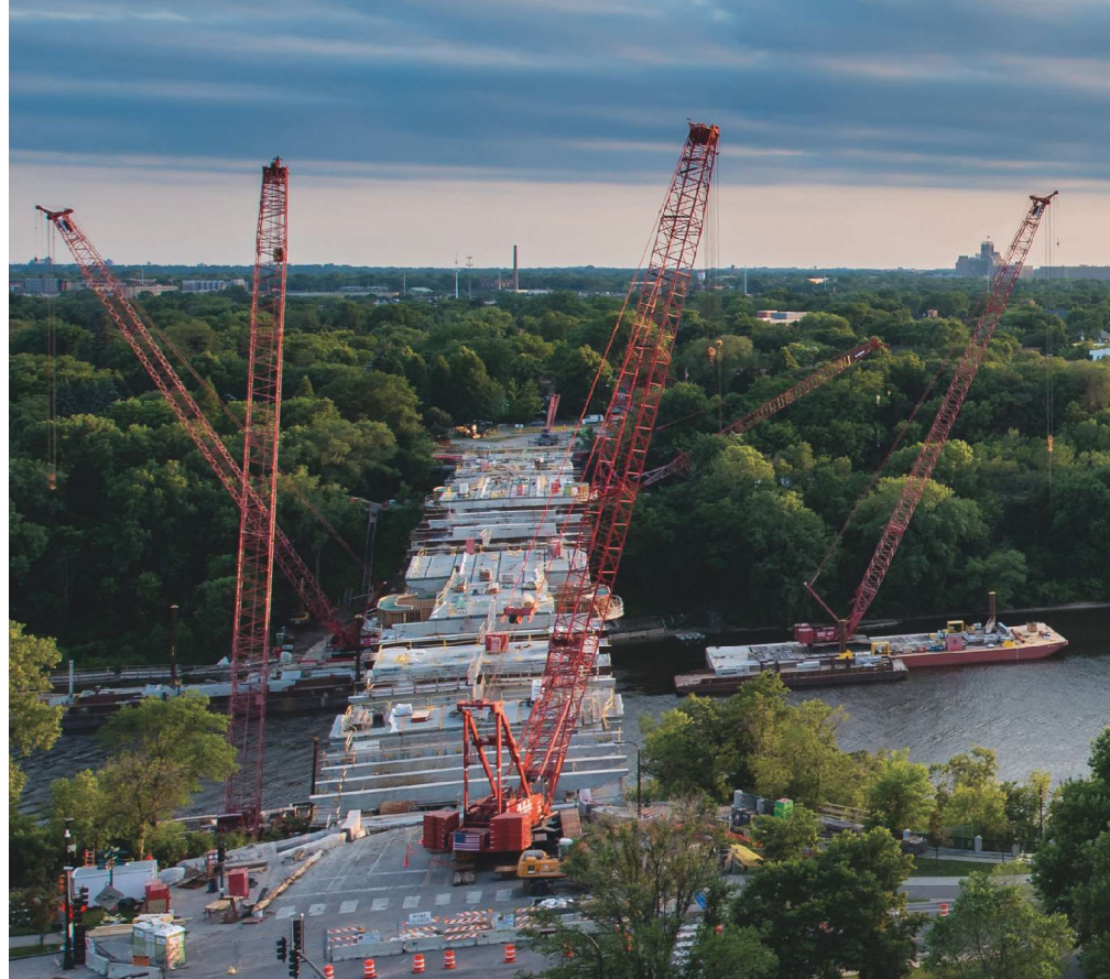
Accelerated bridge construction (ABC) operation.
