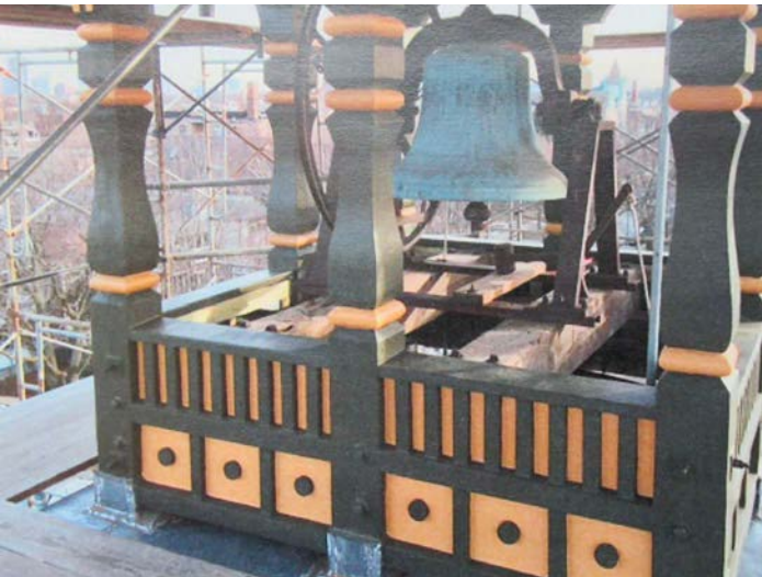
Rebuilt railing (belt-frame) at base of belfry at bell tower.
