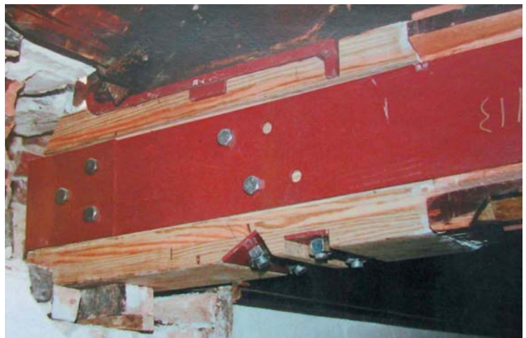
Reconstructed truss end with new preservative treated glulam in position.
