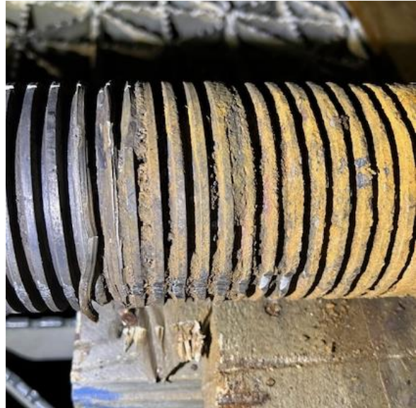
Figure 3: A take-up nut was seized and the threads were damaged when using a hydraulic torque wrench to remove the nut.
