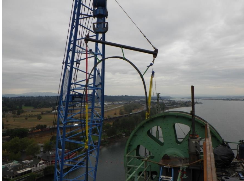
Figure 8: Counterweight rope installation with a crane and spreader beam.
