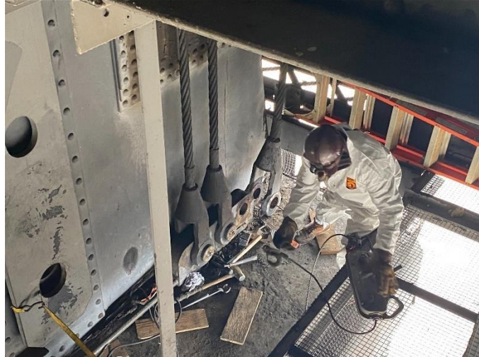
Figure 6: The counterweight end pins are seized and nuts are welded on to remove the pins with jacks.
