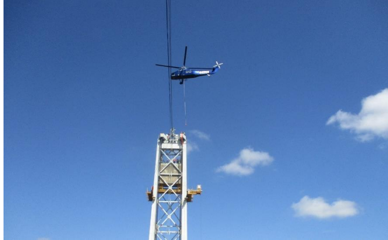
Figure 10: Counterweight rope installation with a helicopter.
