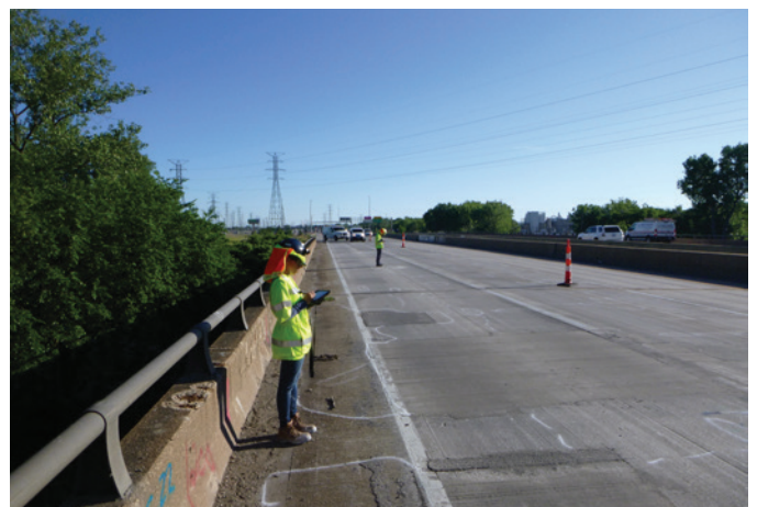
Fig. 3: Bridge Inspection Engineer performing routine inspection of a bridge deck
