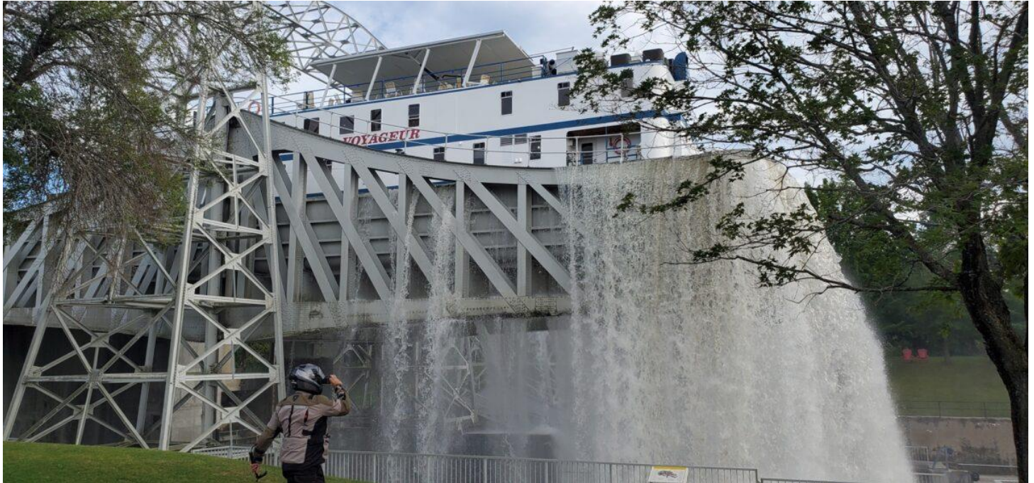
Figure 7 Incident at Kawartha Lift Lock September 3, 2022. (Courtesy of Kawartha 411)
